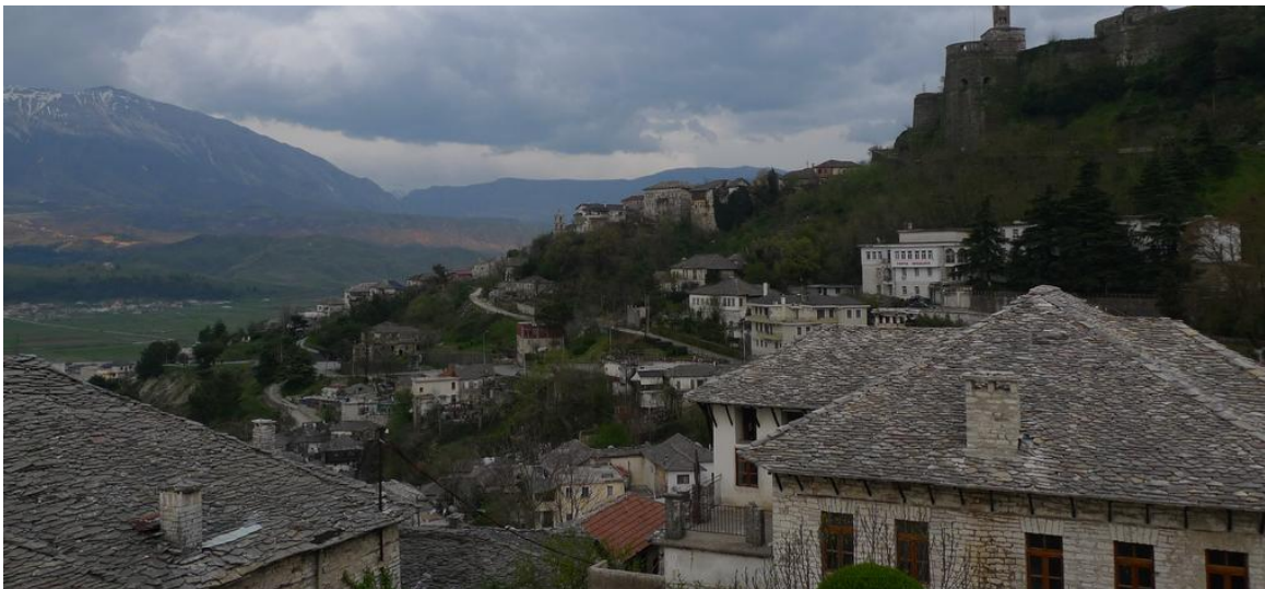
Figure 2: Roof landscape with traditional stone cover in Girokastra, Albania; Source: M. Ripp.
