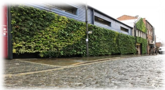
Green walls on business Premises (Liverpool)
